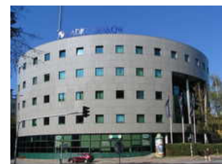
The building of Krakow's radio
