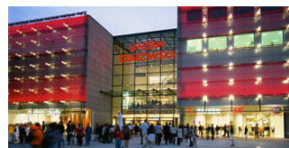
The modern style entrance to Galeria Krakowska
